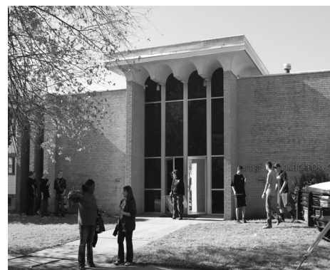
The OZ "extreme makeover" was made possible by individuals and businesses coming together to renovate the lower level of the building.
