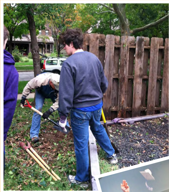
For his Eagle Scout Project, Thomas Spillman and 25 Troop 542 members, parents and friends repaired two sections of broken fence, power washed the patio and furniture, and mulched flower beds.
